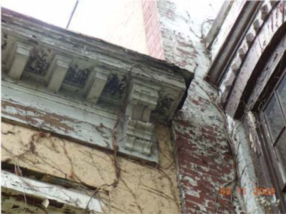
Figure 3 Window and cornice, 1236 New Jersey Avenue
