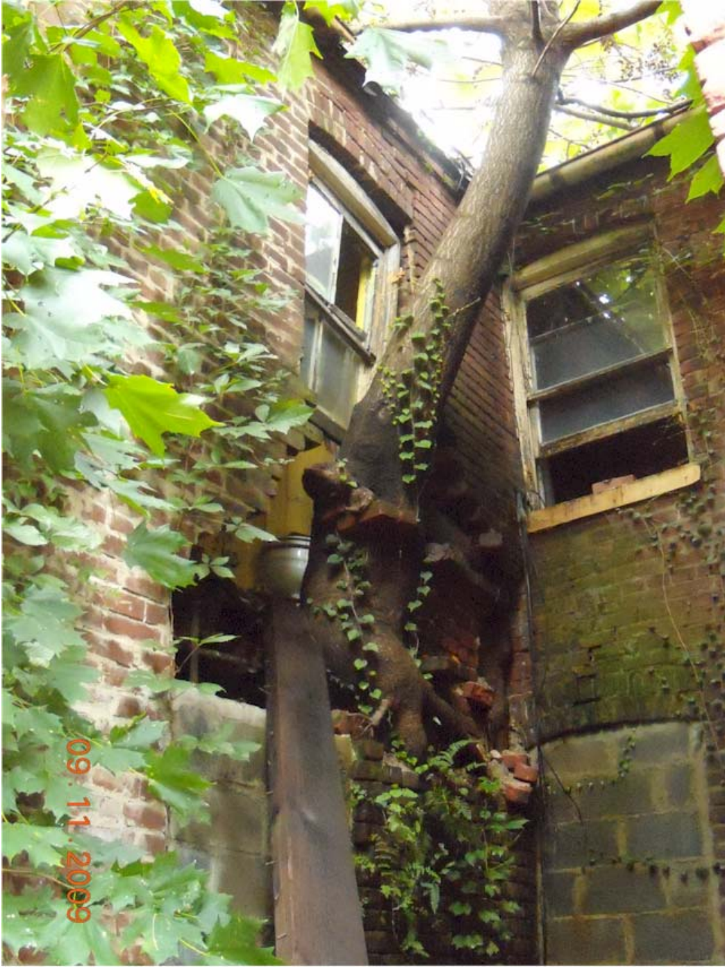
Figure 5 Rear of 1236 New Jersey Avenue
